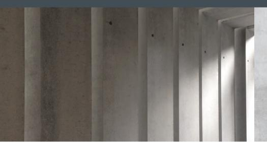
**Phenox NFO 500** is suitable for all smooth, jointless concrete surfaces in accordance with DIN 18202/3, line 5/6 with higher requirements.
